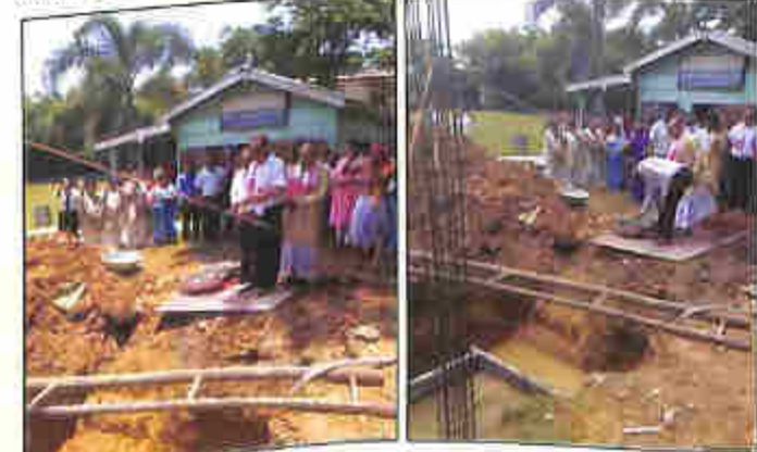
New Building Construction
